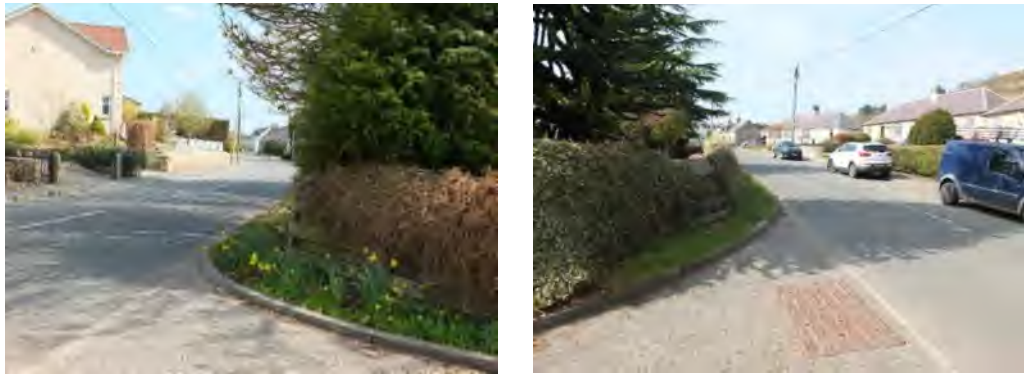
Clear visibility exists to east and west along Leslie Road from a point 2 metres back from the road edge.
