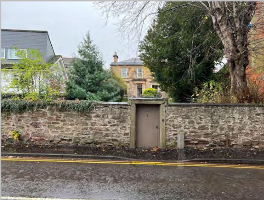
Images 2 and 3: Rose Cottage site frontage with random rubble retaining wall pointed in lime with pedestrian gate.
