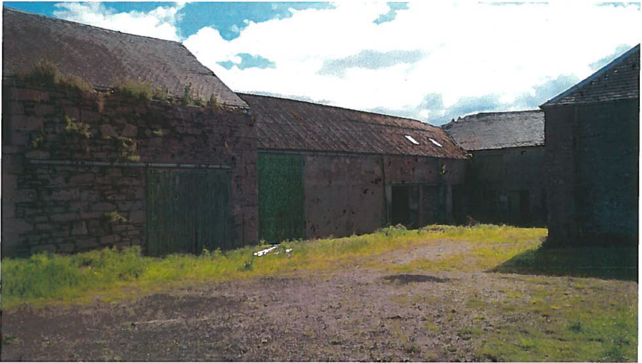
Derelict steading building to SE of site (part owned by applicants)
