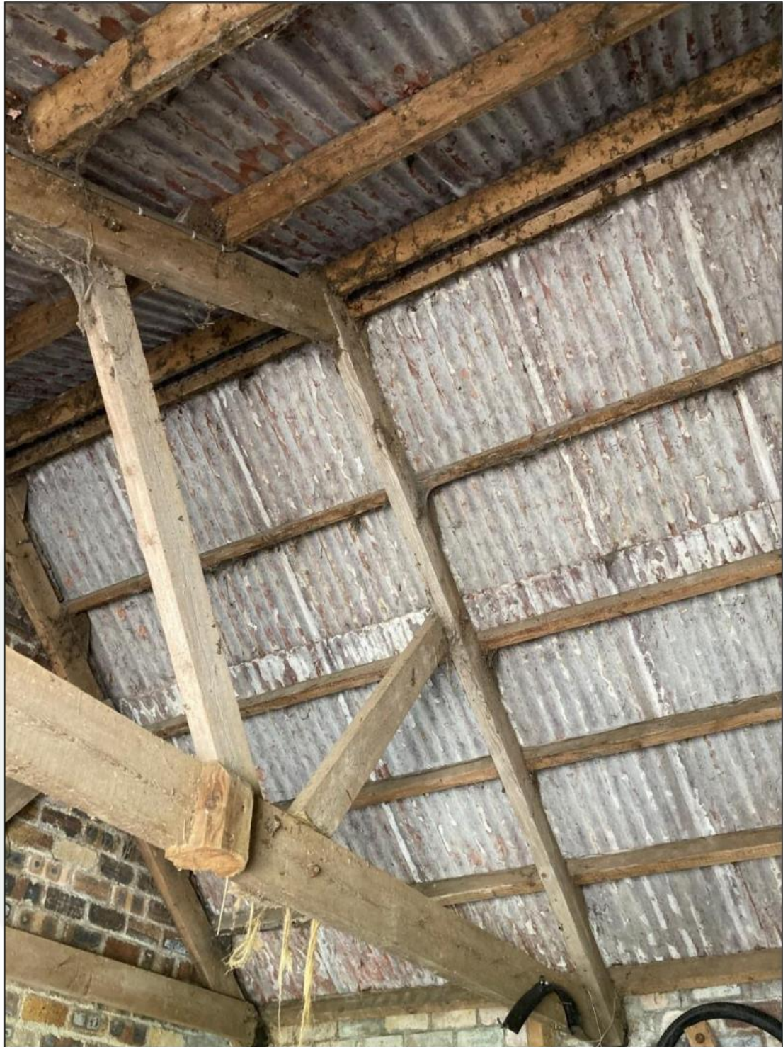
Figure 3. Corrugated metal sheets laid onto wooden joists with no wall or roof cavities present.
