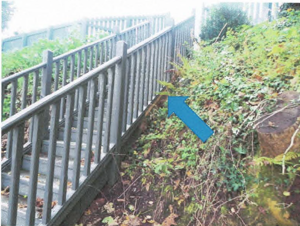
Side view of stairs showing posts, handrail, spindles, treads and stair string. The arrow highlight areas of the structure in need of decoration.
